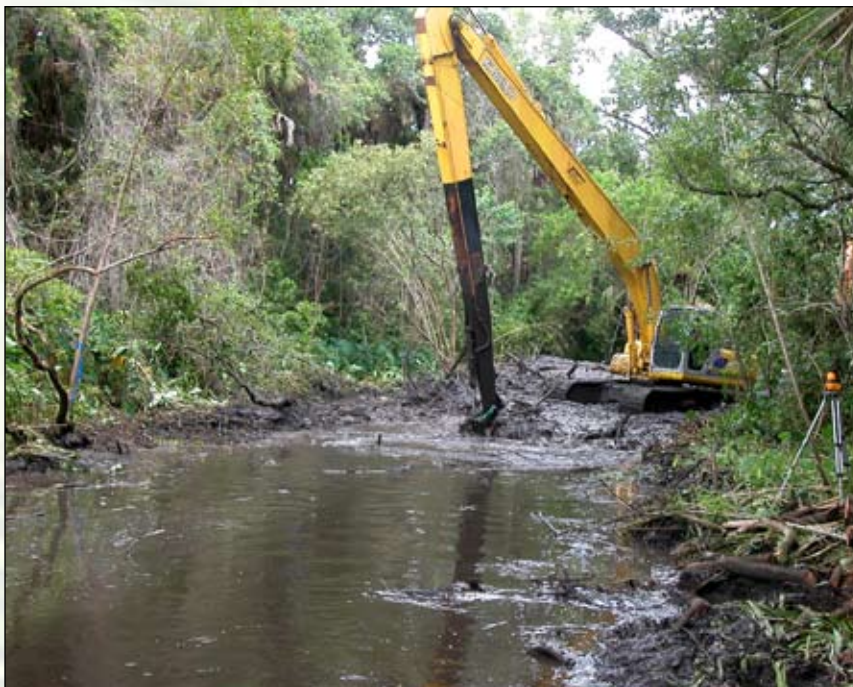
Reconnection of isolated oxbows will improve water quality by decreasing nutrients and suspended solids.
